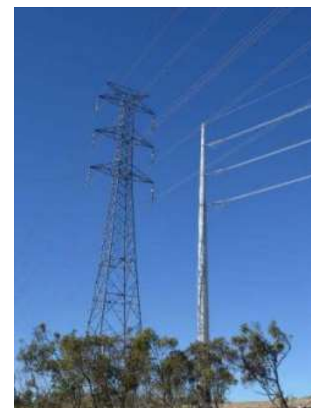
New power pole ready for connection
