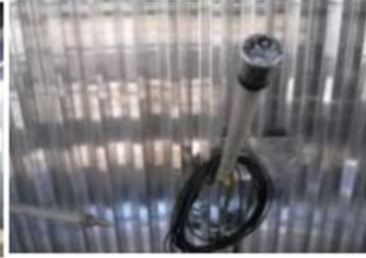
Boiler Tube Leak Sensor Installation
