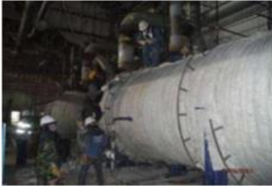
Insulation Installation for HP Heater at STH – Unit 1
