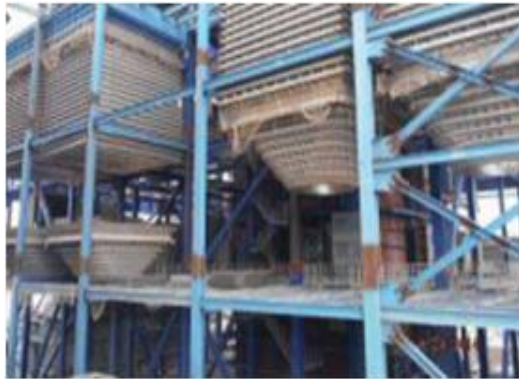
Coal Bunker Installation Unit2
